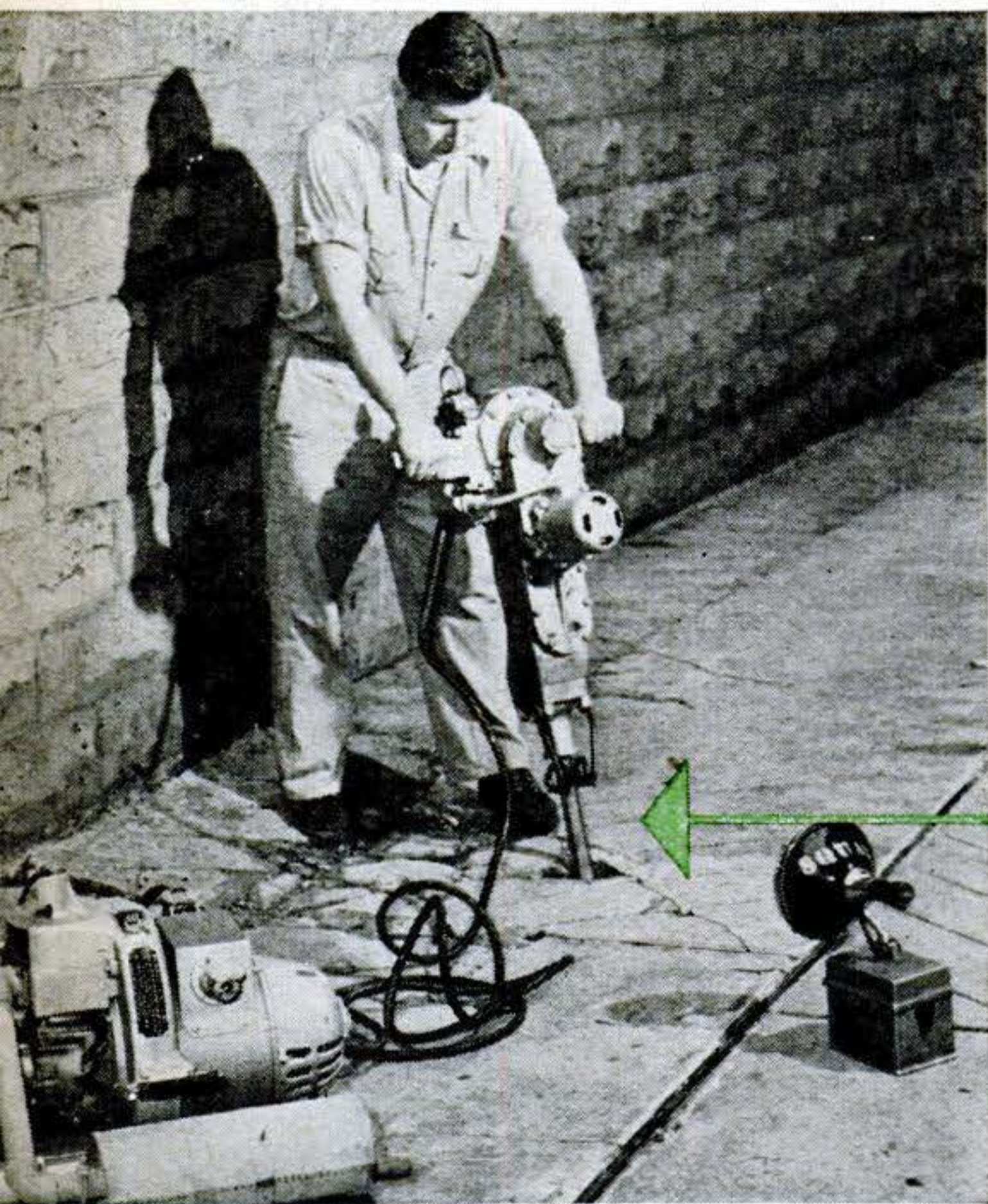
PAVEMENT BREAKER , or air hammer, lets rescuers punch through reinforced-concrete floors in commercial buildings to ventilate basements. Portable generator runs it.
